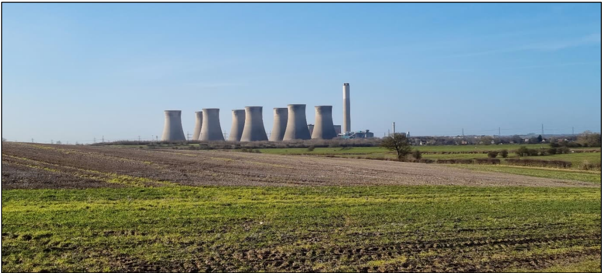
Plate 20 View southwest from the Viking Winter Camp towards Cottam Power Station
