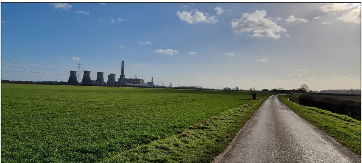
Plate 27 View southeast across the Cable Route Corridor towards Cottam Power Station
